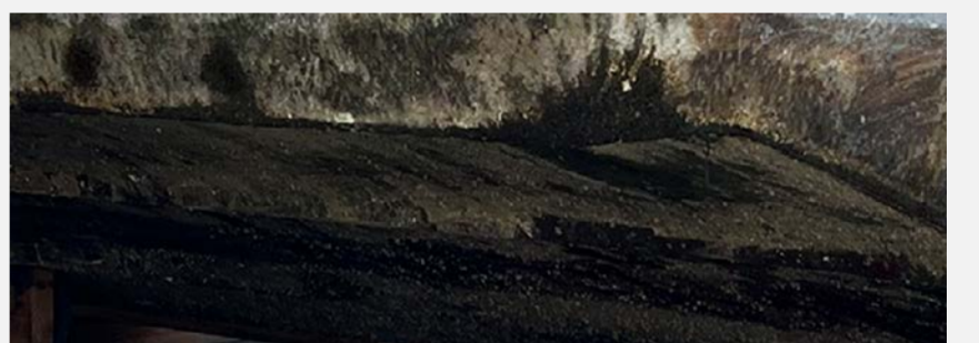
UNPROTECTED PONTOON SHOWING GROWTH
