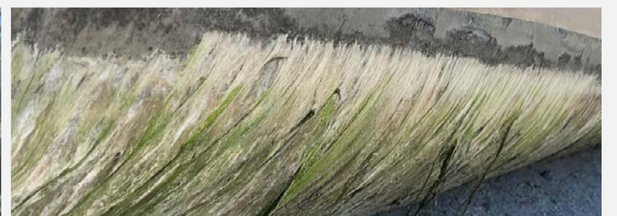
UNPROTECTED PONTOON SHOWING GROWTH
